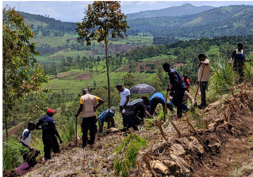
Mentorship team working on connecting water harvesting structures during the in-person support in South Kivu in December 2019. Breakages in berms was a common challenge surfaced during the remote mentorship Phase 1-2, thus the team decided to focus on reinforcing berms and building overflow structures during the in-person support.
